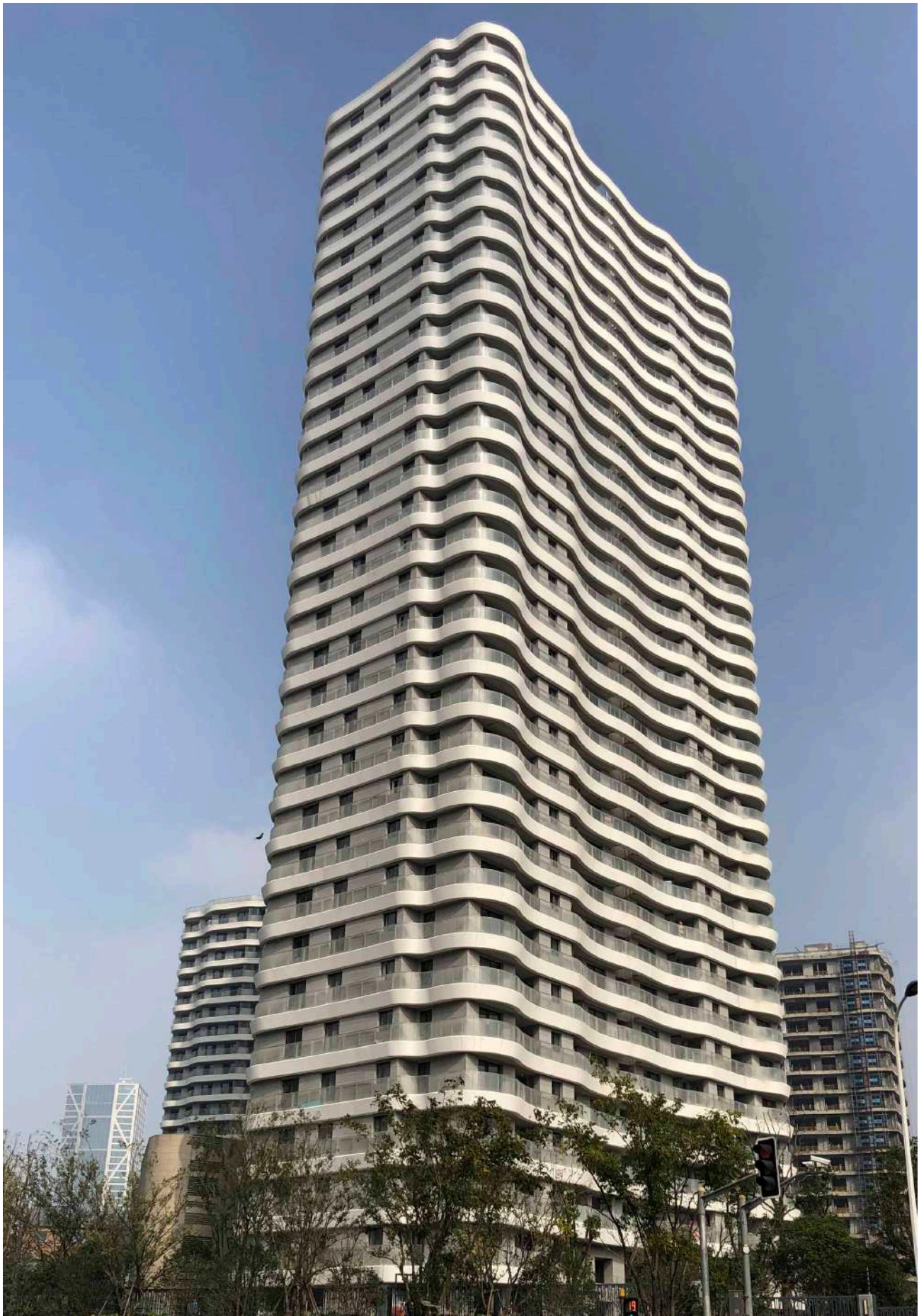
China, Shanghai Nove Masion Residential and office building
