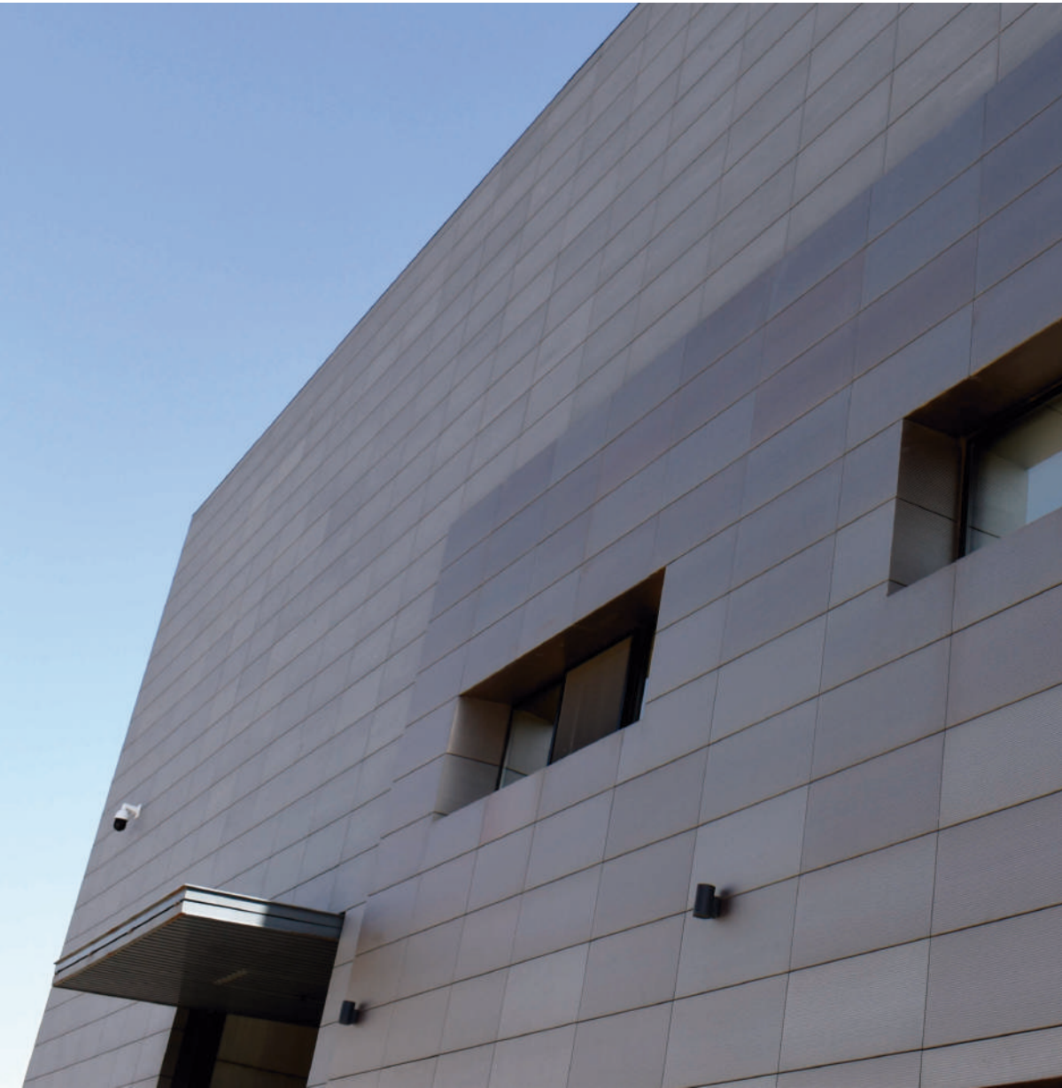
Spain, Toledo Commercial building
